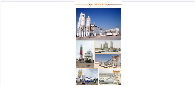
A full-scale view of the stationary plant showing the integration of silos, conveyors, and the central mixing unit.
