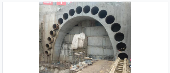
Example of a completed pipe roof tunnel structure.
