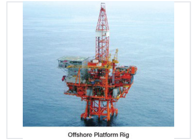
Offshore Platform Rig
