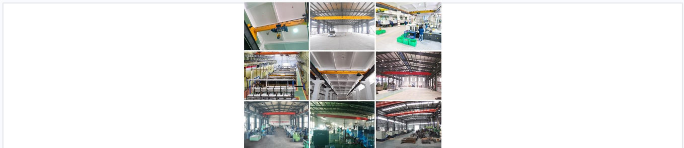
A typical EOT crane installation in an industrial workshop, showcasing the bridge girder and hoist mechanism.
