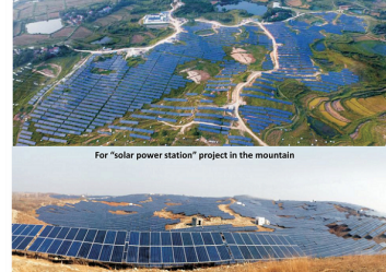
Successful solar power station projects from "QIXING"
